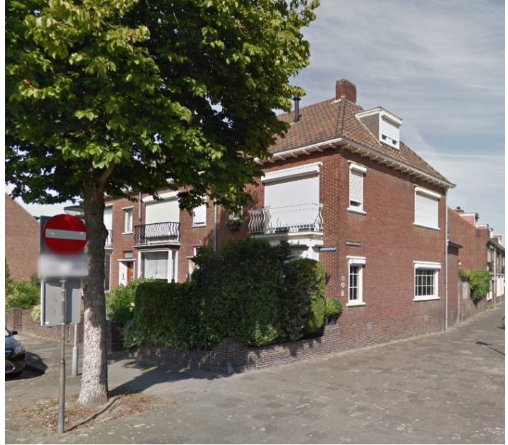
Figure 1. Roll-down shutters in the city of Venlo. Source: Google Maps.
